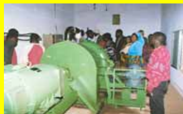
Existing hydro 100 kW at Welela
